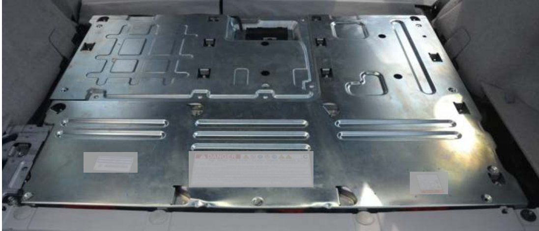
Figure 8 Battery A compartment in cargo area with carpet and molded plastic cover removed
